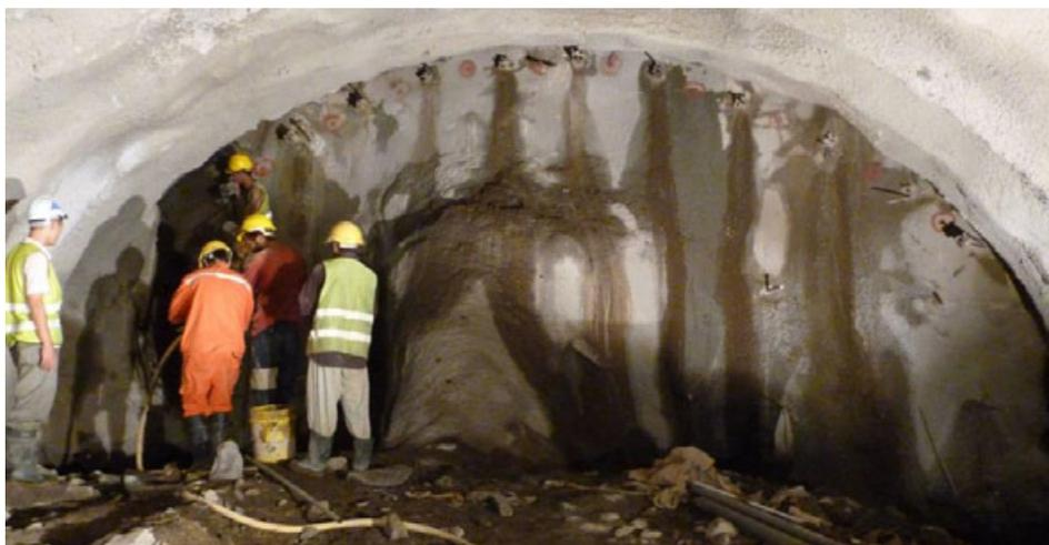
**Figure 18:** Canopy tube grouting at Ch.735 after pneumatic (dry) drilling and tube installation. The photograph shows the release of liquefied *in-situ* mud of the brownish-blackish matrix material from the holes, which is flowing down the face.
