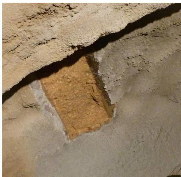
**Figure 11: Spalling of shotcrete at the tunnel perimeter in-between canopy tubes. Radial cracking of the shotcrete at the face and buttress further demonstrated ongoing instability in the face.**
