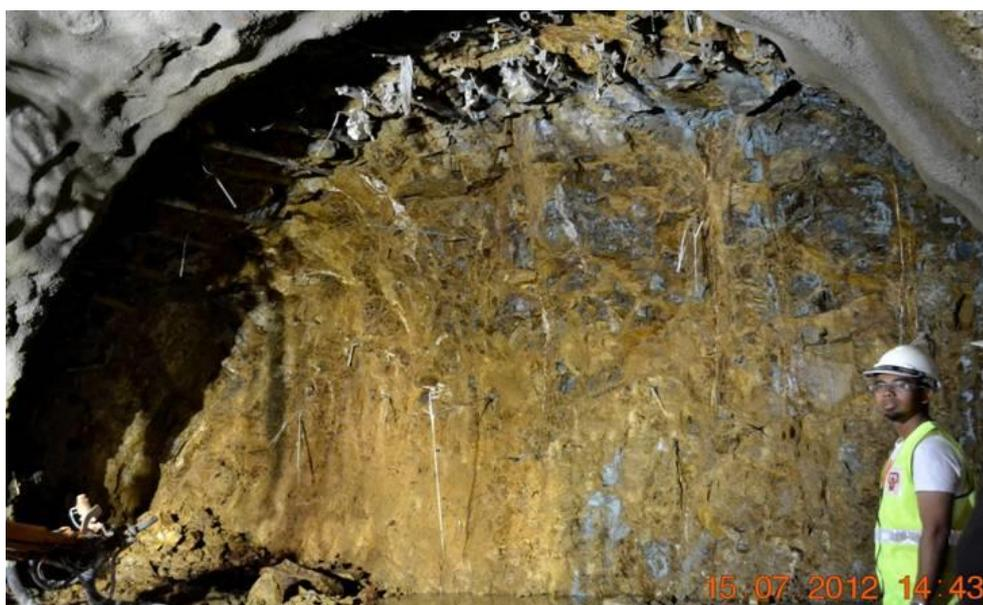
**Figure 6: Tunnel face at Ch. 760 prior to shotcreting and placing of steel set. Cohesive yellowish-brownish matrix material and dark-grey andesite blocks (BiM-rock fc25).**
