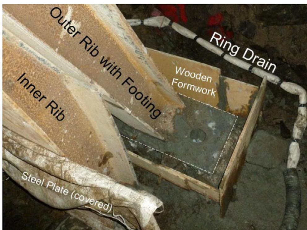
**Figure 9: Details of rib footings prior to shotcrete application. The footing of the outer ribs (highlighted with the dashed white line) stands on aggregate and a wooden formwork was installed before the rib footing pit is filled with grout. A ring drain of wound geotextile is nailed onto the soil to prevent water from the walls entering the excavation pit of the footing. A steel plate is welded on the inner rib in preparation for the installation of micro-piles.**
