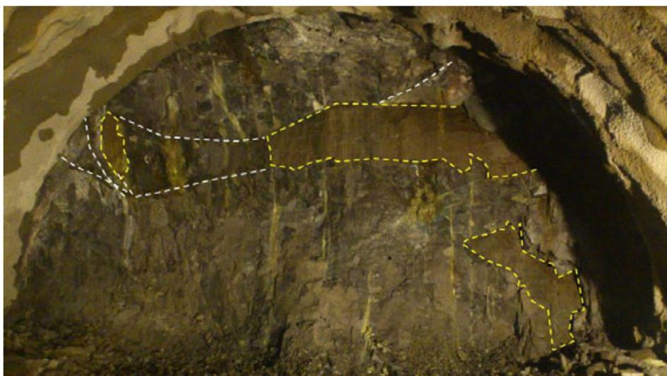
**Figure 19:** The geological conditions got rapidly better once the damage zone was reached. Fractured andesite and lenses or bands of clayey-silty soil at Ch. 722 are exhibited in the tunnel face. The lenses of soil are marked with dashed yellow lines. Some of the lenses were connected with long shear fractures (dashed white lines).
